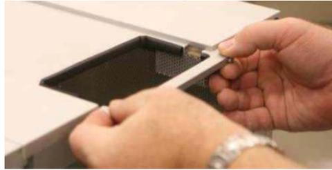
9. Screw in 2 screws to secure the bridge.
